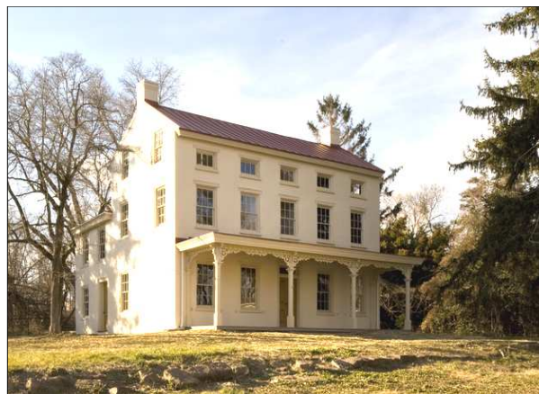
The rehabilitation of Frick's Locks village is complete! Photograph by Frens & Frens, Restoration Architects.
