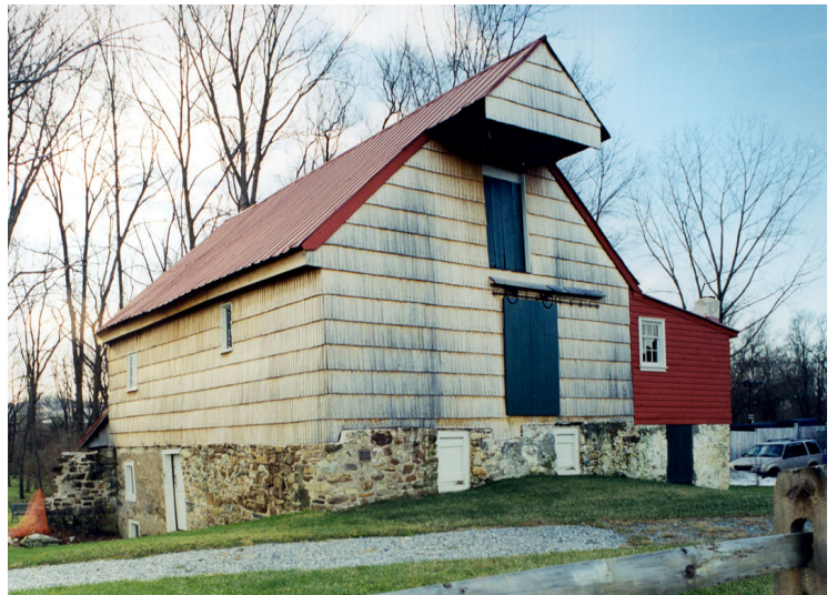
Thomas Mill, 1744, after award-winning exterior rehabilitation
